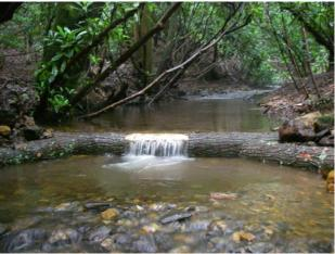
Before and after photos of Gurley Creek representing a typical brook trout stream on Chattahoochee National Forest. This log structure increases stream depth in the plunge pool, increases pool depth upstream of the structure, and provides cover through the addition of large woody debris. Photos were taken by Leon Brotherton (GA-DNR) in July 2009.
