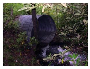
deterioration with water flow around and under the pipe. The pipe will be replaced by a bottomless arch. This will connect approximately two miles of upstream habitat in Bryant Creek with two and a half miles of downstream habitat in Bryant Creek and Pretty Branch.
