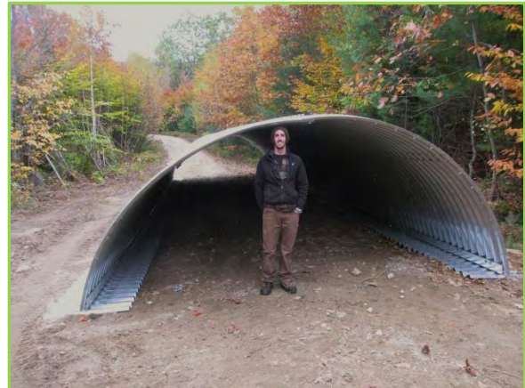
Figure 3: Ash Bog Stream culvert. Photo by Dan Grenier.
