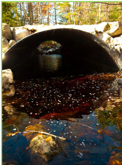
Figure 7: Ash Bog Stream culvert outlet following construction. Photo by Nancy Sferra.
