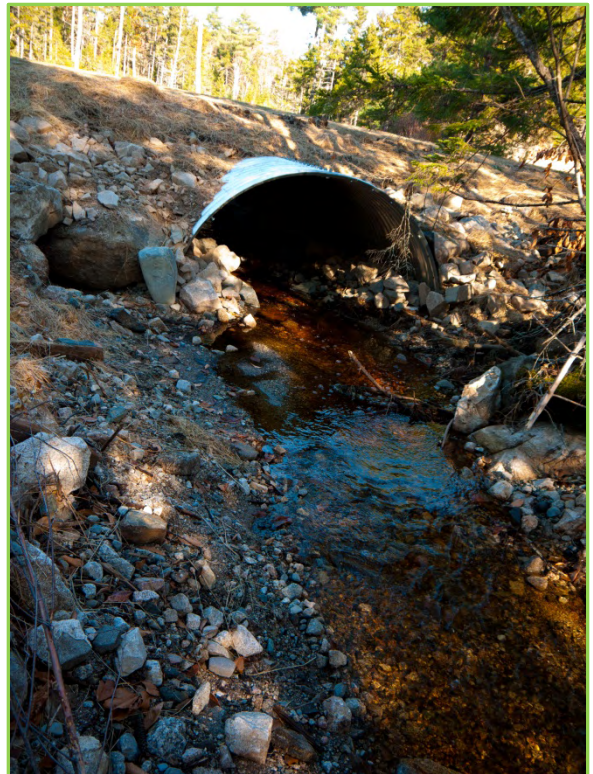
Figure 14: Black Rock Brook downstream following culvert installation. Photo by Nancy Sferra.
