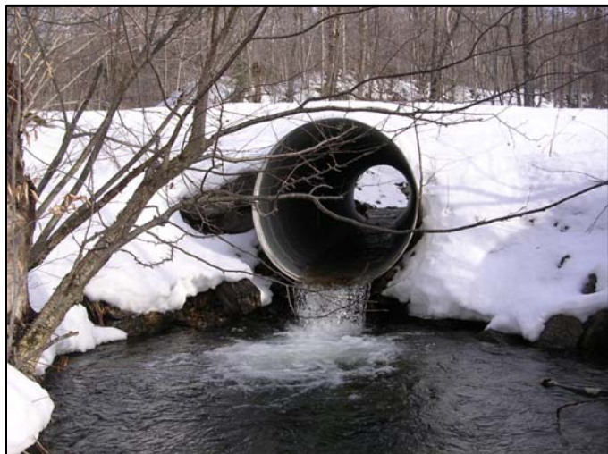
Culvert causing a passage barrier to brook trout in Stevensville Brook (Courtesy Chris Smith- USFWS)
