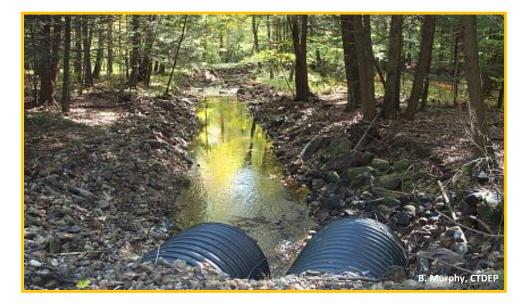
Figure 2. Photograph illustrating skewed alignment of culvert outlet directing high stream flow regimes into streambank and downstream area of past channelization.
