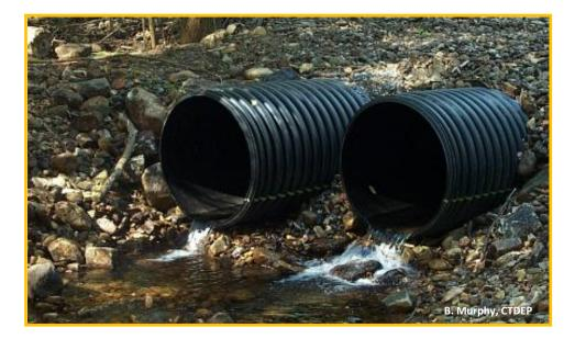
Figure 1. Photograph depicting outlet of twin culverts perched above streambed. Improper culvert installation blocks and prevents upstream passage for the wild brook trout population.
