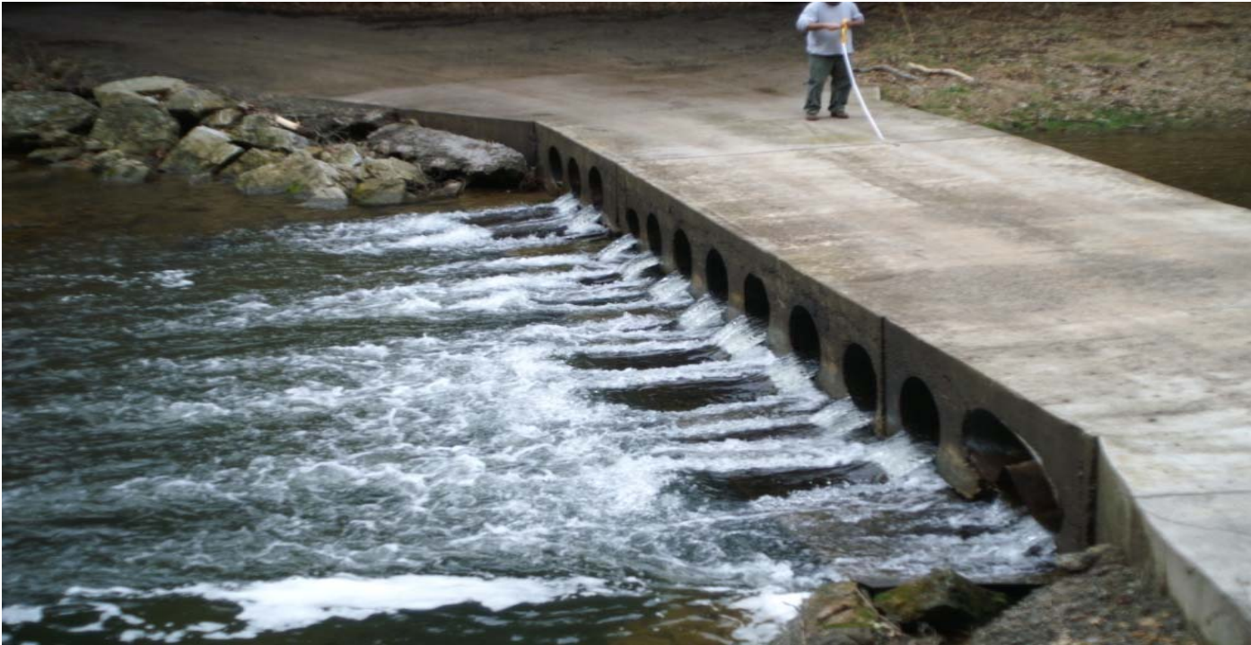
Figure 1: Propst 's low water bridge, typical of three fish passage obstructions in the watershed.
