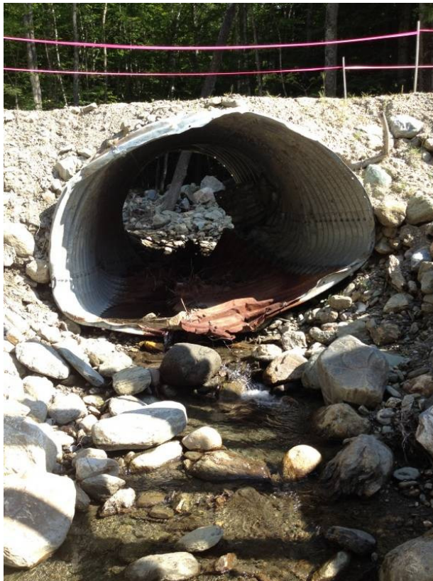
Nason Brook culvert at Woodlawn Cemetery (Greg Russ, White River Partnership)
