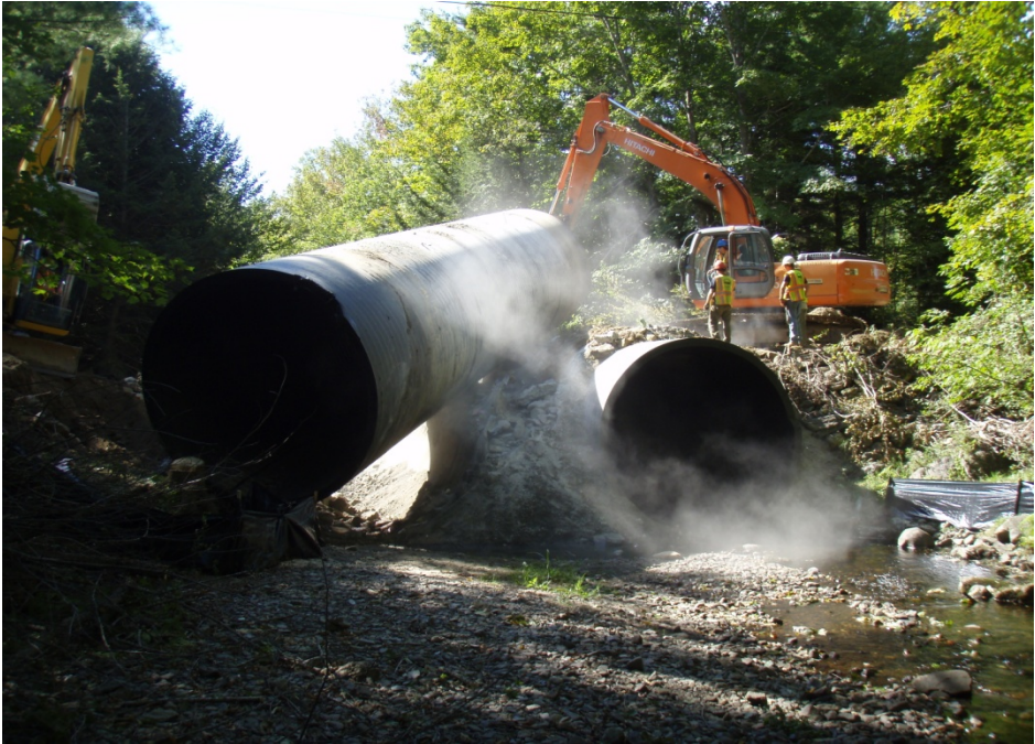
First pipe removed.
