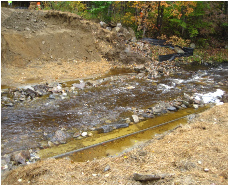
Both Footers Installed.
