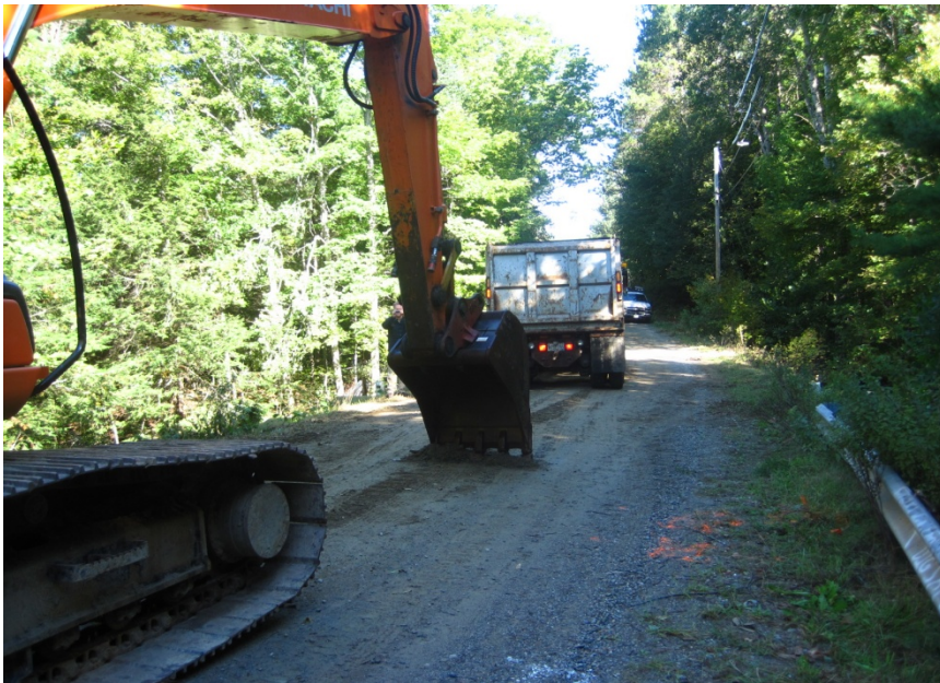
Beginning of Excavation
