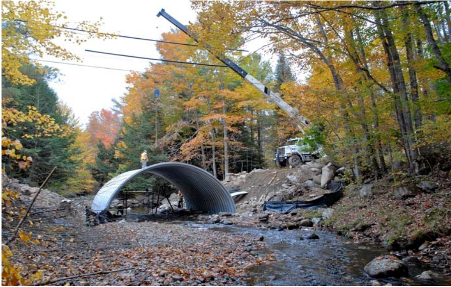
Placement of First Section
