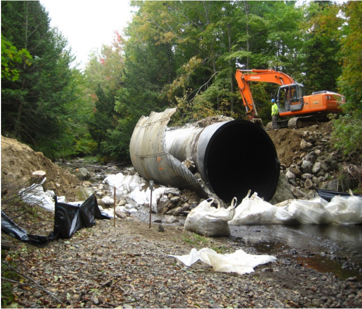
Water Passed Around Second Pipe.
