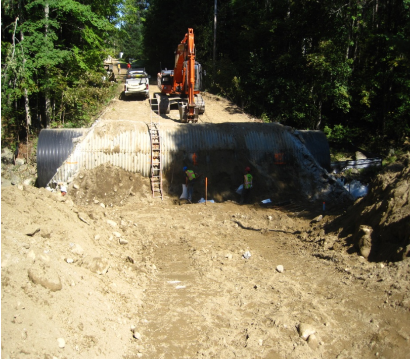
First pipe exposed.
