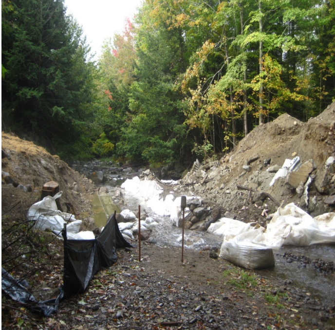
Both Pipes Removed—Note footer
