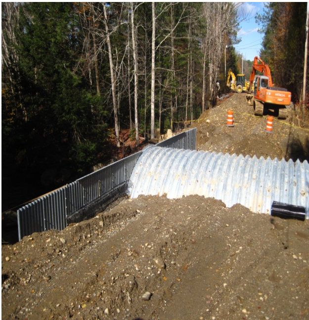
Headwalls Complete—Fill Placement
