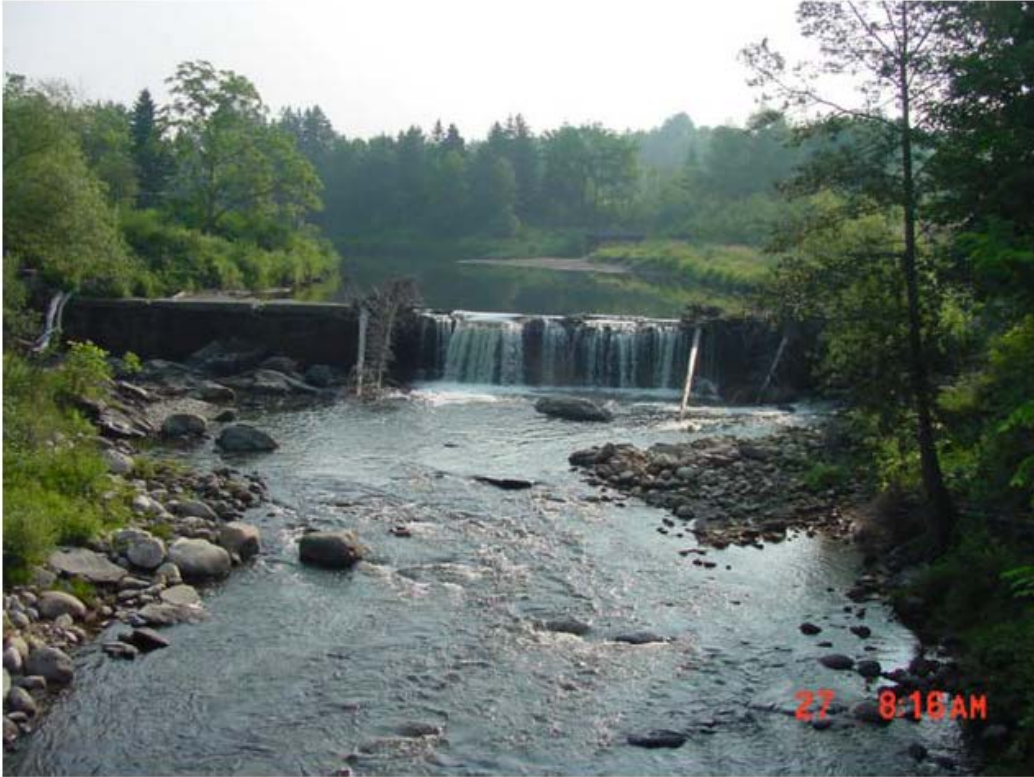
Looking upstream at the East Burke dam, East Branch Passumpsic River.
