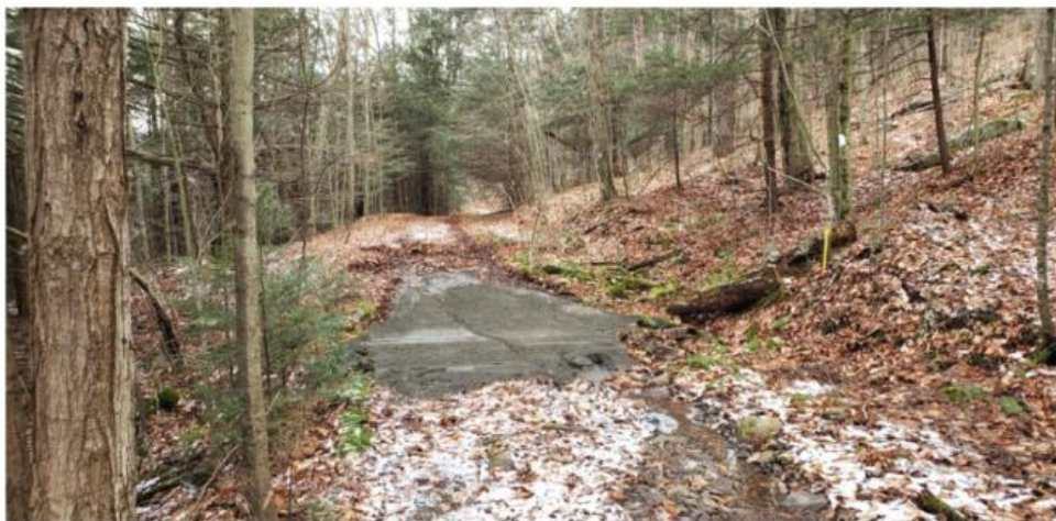
Figure 4 Limestone applications outside of former Lake bottom to increase spring seep pH levels.
