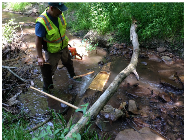
Notched cross-log in downstream former impoundment
