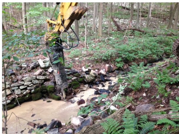
Removing jack dam between two former dams
