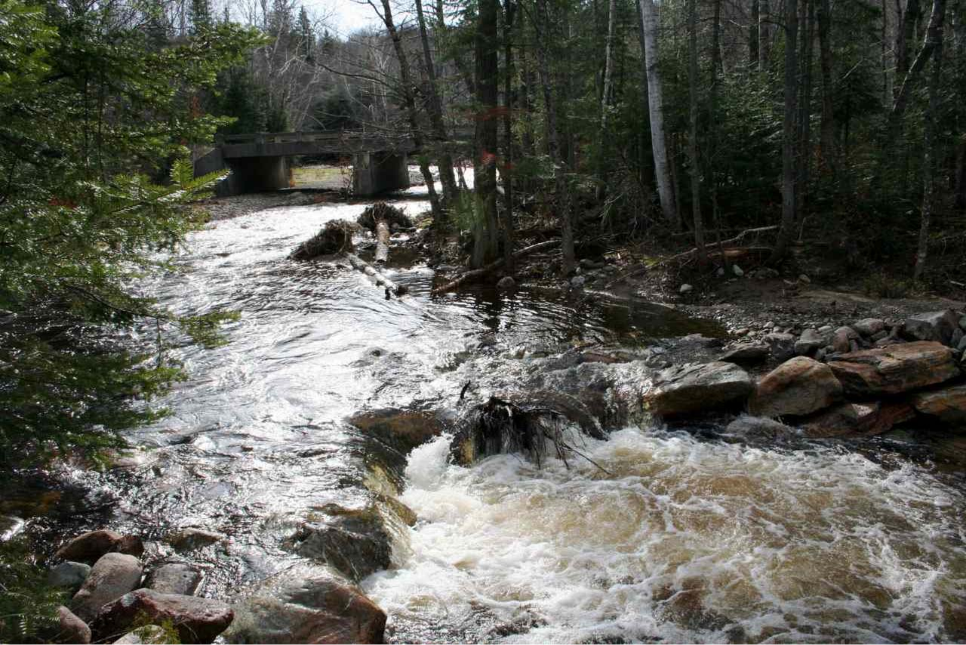
Rock Weir Sunday River
