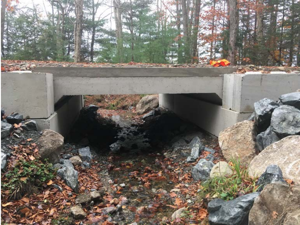
3. After inlet looking down stream
