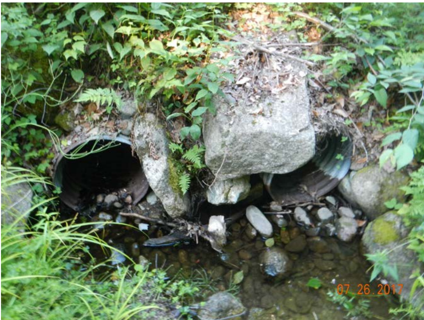
2: Before: culvert inlet
