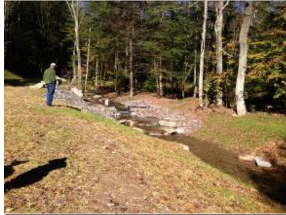
Photo 6 – Completed construction on Rt Br Wetmore Run. credit: PFBC
