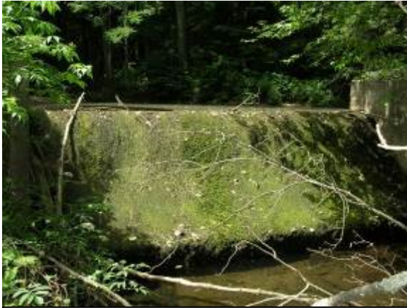
Photo 1 – looking upstream towards Right Branch Dam. credit: PFBC
