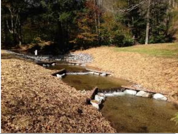
Photo 5 – Completed construction on Wetmore Run. credit: PFBC
