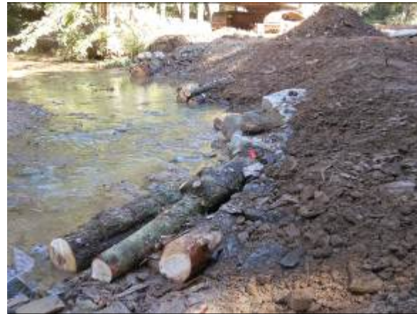
Photo 8 – Log vanes constructed to decrease pressure on the banks. credit: PFBC
