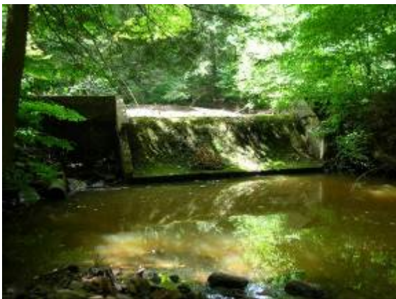
Photo 3 – looking upstream towards Left Branch Dam. credit: PFBC
