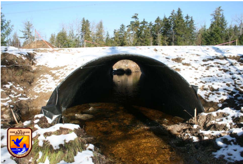
Looking Downstream to the new 12 ft wide Open Arch on Knox Lake Outlet Stream . Oct 31, 2011
