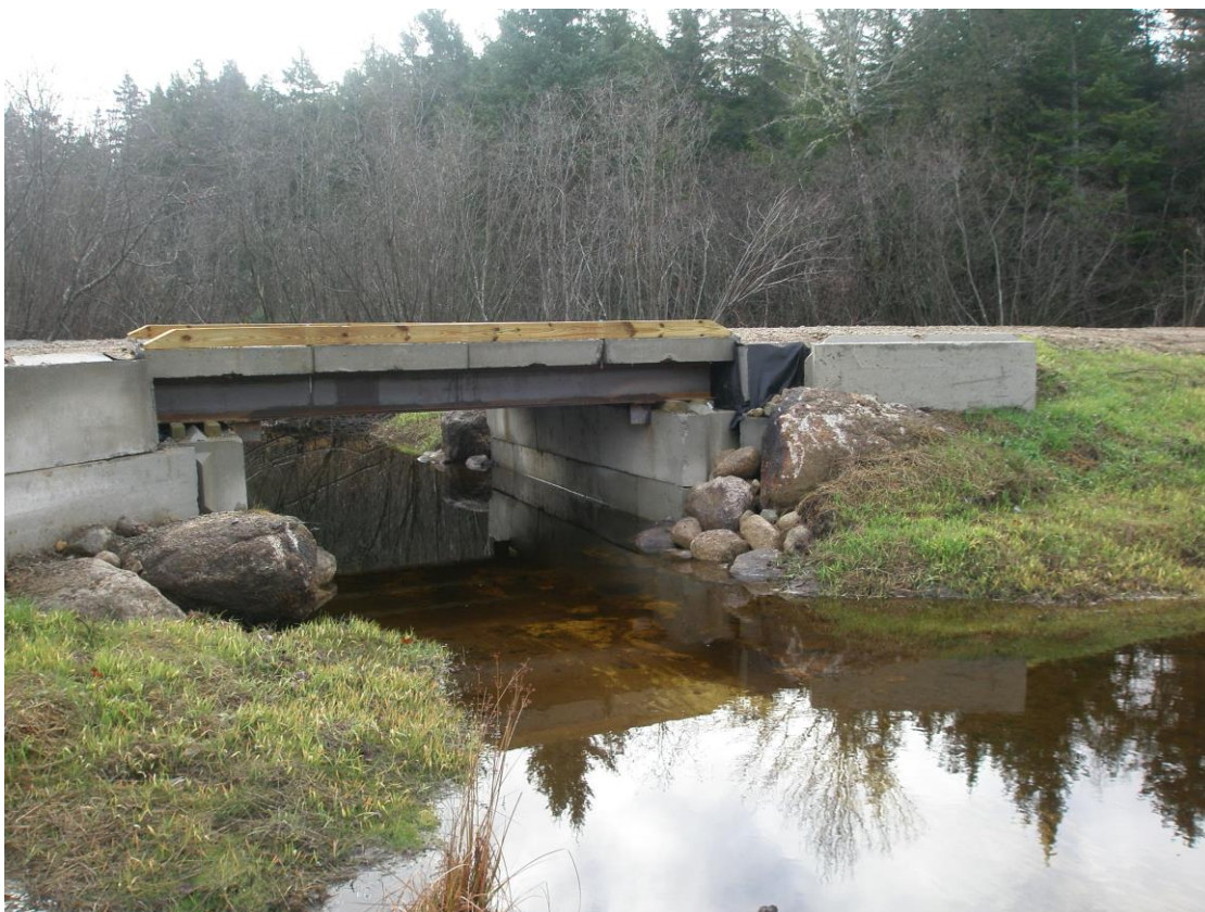
Concrete-decked bridge installed at Towers Brook crossing.
