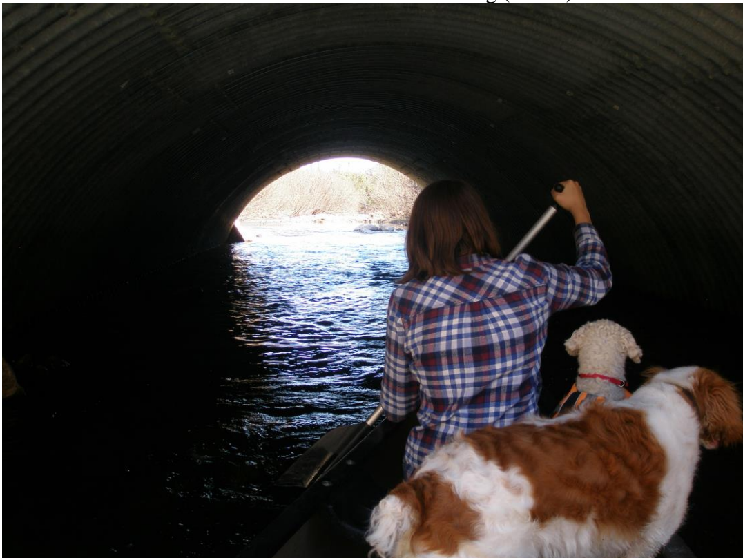
Paddling a canoe through Grand Lake Brook 20' arch culvert (after).
