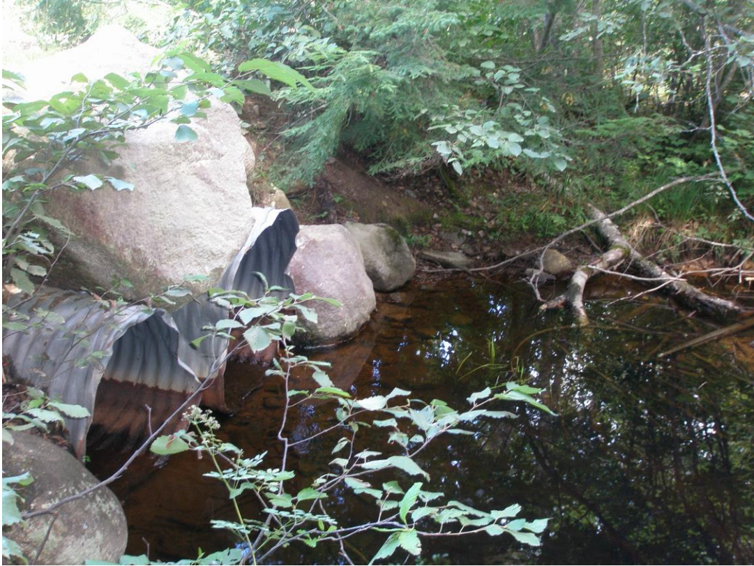
South Branch of Little River before restoration: downstream.
