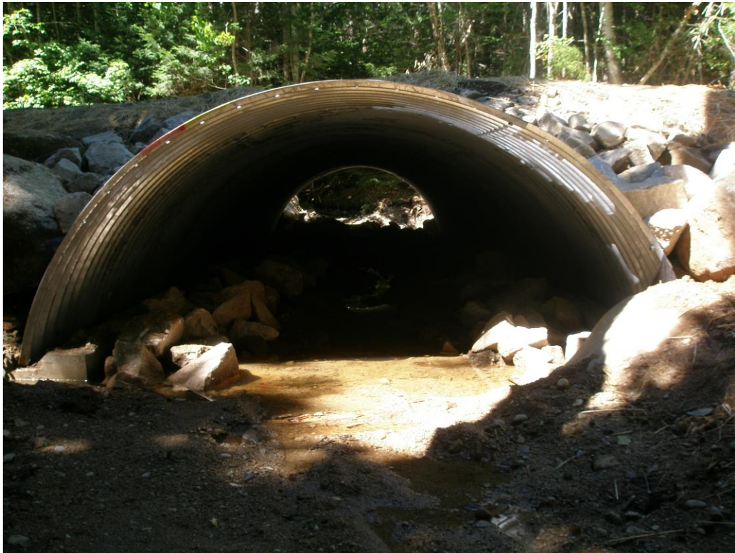
Fourth Lake Trib. after arch culvert installation during 2016 drought.
