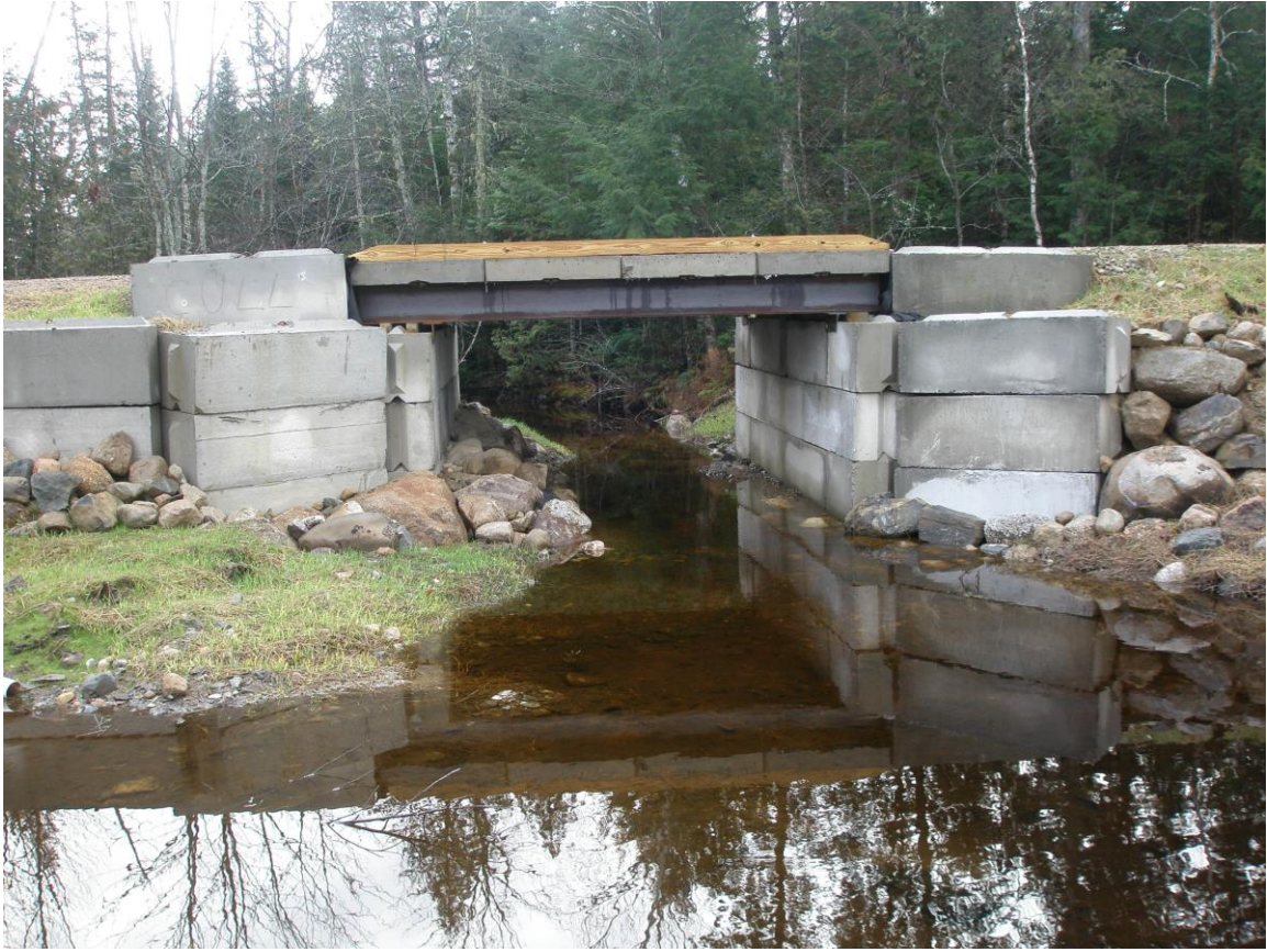
Concrete-decked bridge installed at South Branch crossing.
