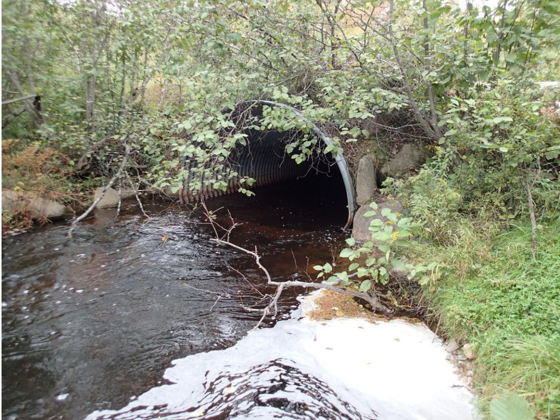
Outlet of Grand Lake Brook crossing (before).
