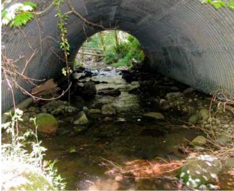
Figure 3. Example of a Well Designed Road-Stream Crossing
