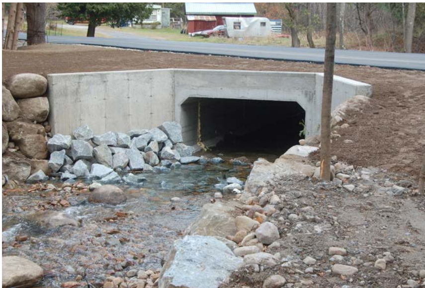
Figure 7. Upgraded Culvert on Lewis Brook
