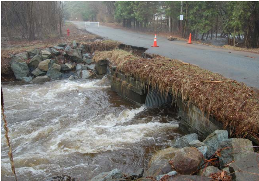
Figure 6: Original Culvert on Lewis Brook
