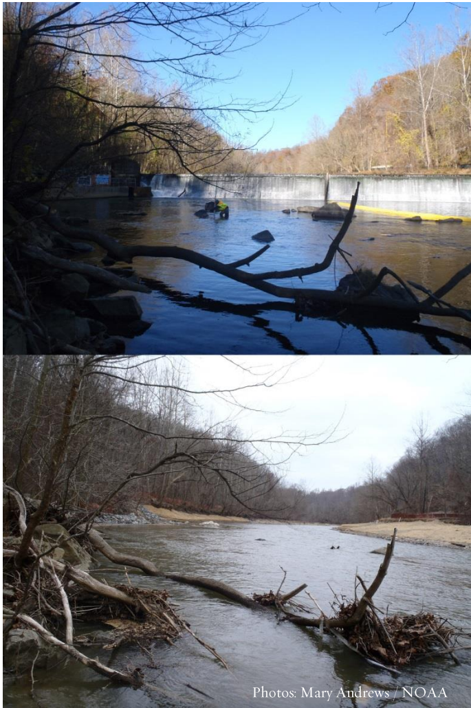
Figure 4-4: Simkins dam on the Patapsco River, before and after its removal in 2011
