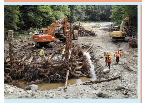
Large photo: Dr.Gubernick (USFS) did a great job showing us how to build the Engineered Log Jams (ELJ) and they are massive! While digging the upper ELJ (3 total) we intercepted a groundwater spring. 48F (9C) water is now flowing into the 6 foot pool associated with this ELJ. No Pools were previously in project area- we now have 3! - Scott Craig, USFWS - Maine FWCO.
